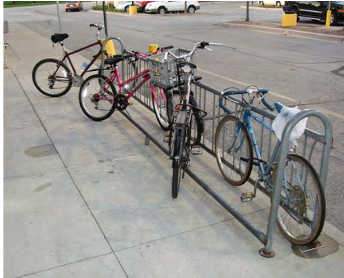
Top: This rack type does not allow for secure or efficient bike parking and should not be utilized.
