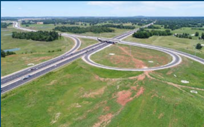
The new I-65 interchange and connector road, near Oakland. Photo courtesy of KYTC.
