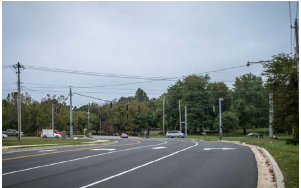
The completed Phase I Smallhouse Road widening project at the intersection with Campbell Lane.
