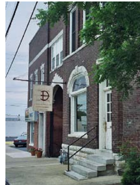
Appropriate sign locations and types are board over storefront, hanging sign over storefront, on awning or on window. Above is an example of a hanging sign and below is an example of a sign on an awning.
