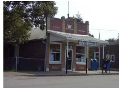
This commercial structure in Oakland has a false front and a gable roof. DEFINITION: A "parapet" is a low wall or protective railing; often used around a balcony or balconet, or along the edge of a roof. Info: Old House Dictionary .
