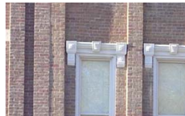
Window hoods and surrounds are architectural features that help give an historic building its unique character.
