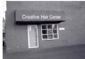
Narrow plastic awnings are incompatible with the materials of historic commercial buildings, and provide no weather protection benefit. Image & Info: KY Streetscape Design Guidelines for Historic Commercial Districts .
