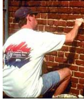
Before 1920, most mortar was composed of a mixture of lime and sand. This composition allows for expansion and contraction of the joints in hot and cold weather. Mortar used to repoint buildings built prior to 1920 should be of similar composition and should match the original color. This early 19th century building is being repointed with lime mortar. Photo: Travis McDonald.
