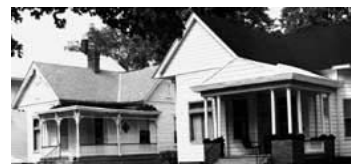
When aluminum was installed on the house on the right, the barge boards, scrollwork, columns, and railings were removed. The distinctive shingled gable and attic vent were covered, further compromising the building's architectural integrity. Photo: NPS files.
