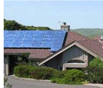
This solar panel is inappropriate but would be allowed on the opposite rear slope of the roof.
