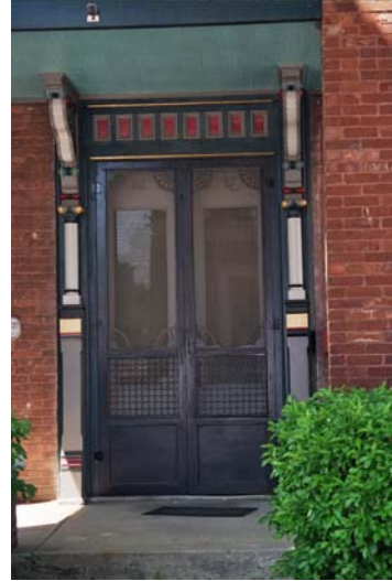
The house at 1149 State Street retains its original screen doors. It has been painted to match the colors of the entrance.
