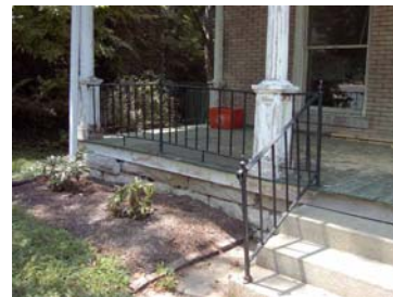
This wrought-iron porch railing is not original and should not have been added to this 1906 house. New owners have since removed it.
