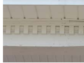
The eaves of this home have been covered with vinyl siding, creating a sharp contrast between the original wood dentil molding and the synthetic material.
